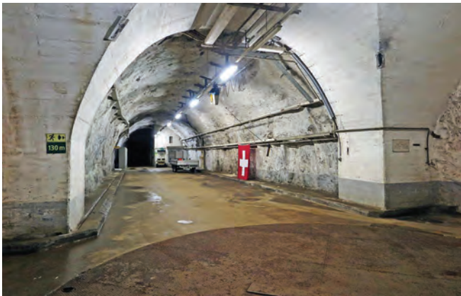
Fort Furggels: The lorry turntable at the end of the main access tunnel into the fort. Photo Clive Penfold
